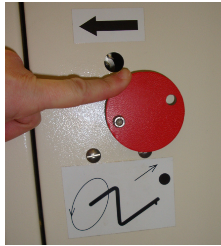
Emergency Crank Switch
